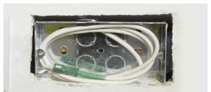
Above - Single ended internal fibre cable Below - Connectorised end of cable coiled in back box
