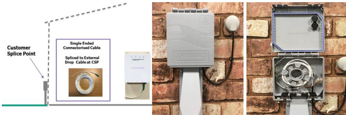
Figure 2 – Customer Splice Point Illustrations
