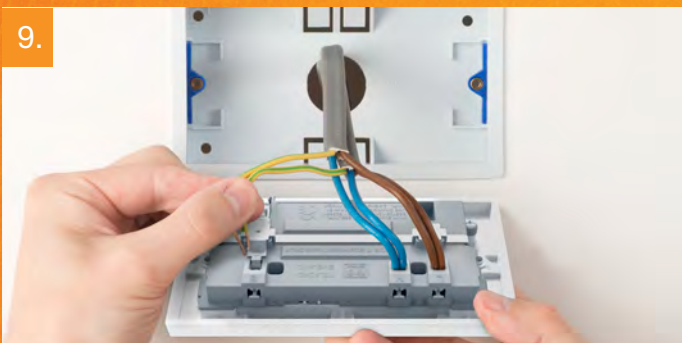
9. Place the blue wire(s) into the neutral terminal, brown into the live terminal and green/yellow into the earth terminal. The terminals on the socket are colour-coded to help locate the correct one.
