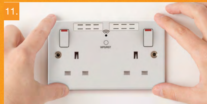
11. Gently press the socket back into place over the mounting box. Take care not to trap any wires between the wall and the socket.
