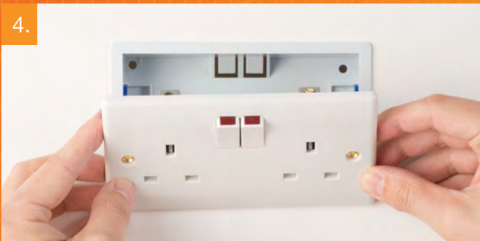
4. Gently ease the socket from the mounting box to show the wiring.
